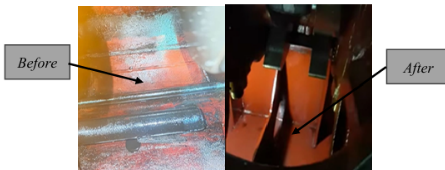
Gambar 7. Cleaning sump tank
