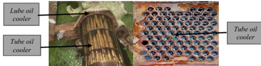
Gambar 10. Tube Oil Cooler Bocor
